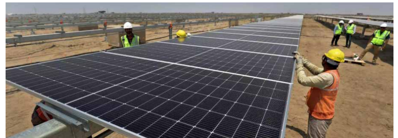
Ongoing work for 3 GW solar power plant in Rajasthan
